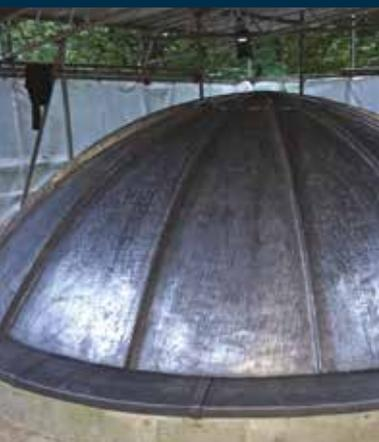
Restoration of Rotunda, including recreating the dome in green oak, adding ventilation and lead covering; lathing and plastering of roof structure with traditional lime putty; entrance gates and circular glass eye.
